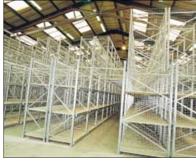
Longspan shelving under construction.
